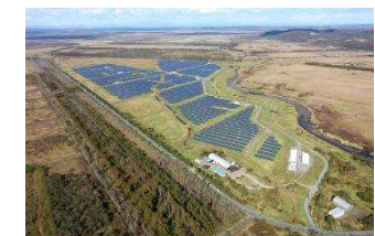
Overall view of the power plant
