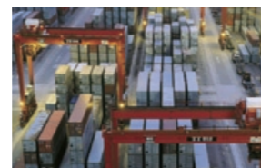
Hybrid transfer cranes
