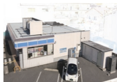
The PV-EV System installed at the Lawson convenience store in Kisshoin Satominami, Kyoto
