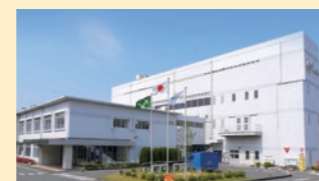
Exterior of GS Yuasa Energy
