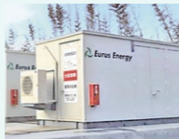
External view of lithium-ion storage battery facility
