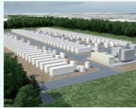
Chiba Refinery, Osaka International Refining Company, Limited
