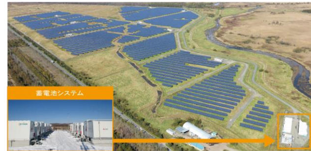
Lithium-ion battery system at a solar power plant in Toritouchigenya, Kushiro-cho, Hokkaido Prefecture
