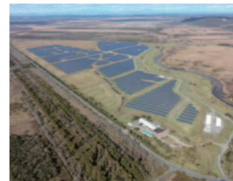
Overall view of Kushiro Toritoushi Wildland Photovoltaic Generation Plant
